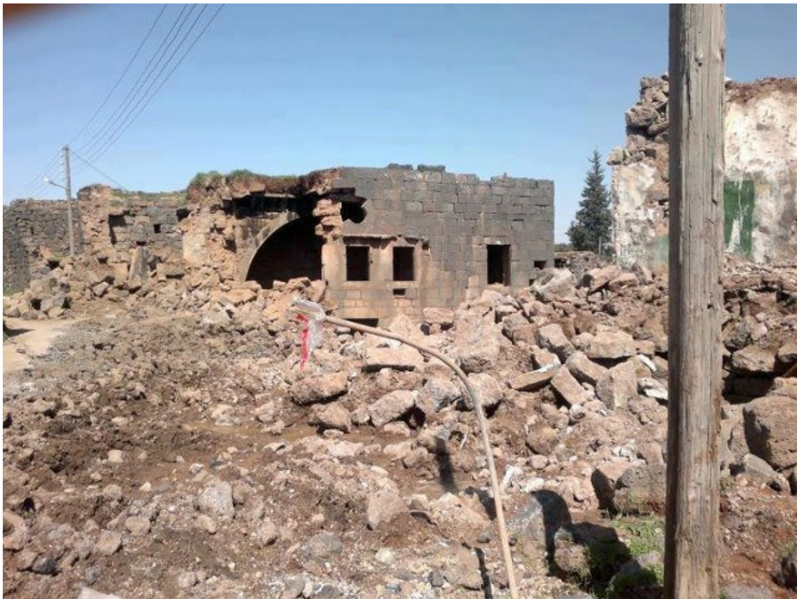
Figure 24: Photo of a heritage house in the North District, allegedly destroyed by the Syrian military 152
