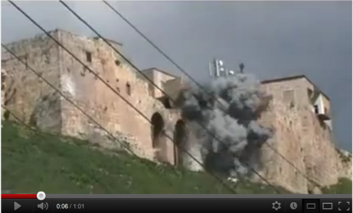
Figure 20: Shelling damage to citadel (15 March 2012) 139
